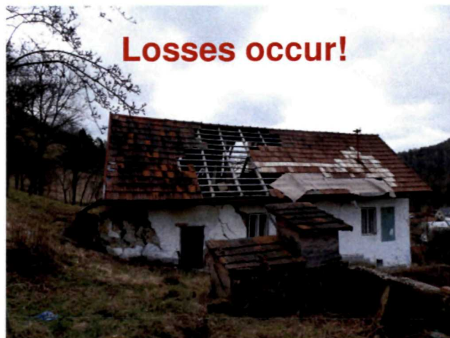
Fig. 1.3 Graphic depiction of the landslide risk assessment methodology (modified according to Alexander, 2002, in Petrydesová, 2012). Photo of destroyed house in the Červený Kameň village, Liščák, 2013
