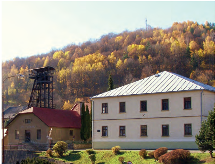
Fig. 3.12 Ferdinand Shaft in Kremnica
