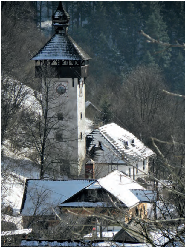
Fig. 3.9 Knocking Tower in Banská Hodruša
