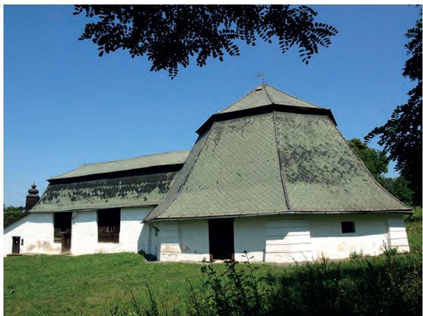
Fig. 3.23 Leopold Shaft – house of winder for the removal of mine water, Slovak technical museum Košice – exposition Solivar Prešov
