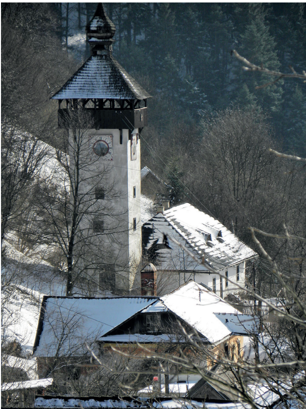
Fig. 3.9 Knocking Tower in Banská Hodruša
