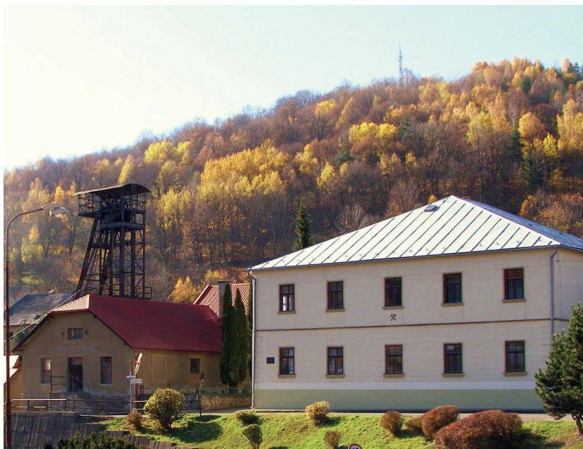
Fig. 3.12 Ferdinand Shaft in Kremnica
